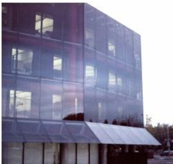
Figura 2.7 - Briarcliff House, Farnborough. Fonte: SAELEN, 2002
