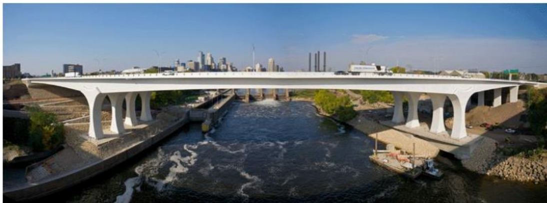
Figura 1.4 – Ponte Saint Anthony Falls. Fonte – Branco, 2013.
