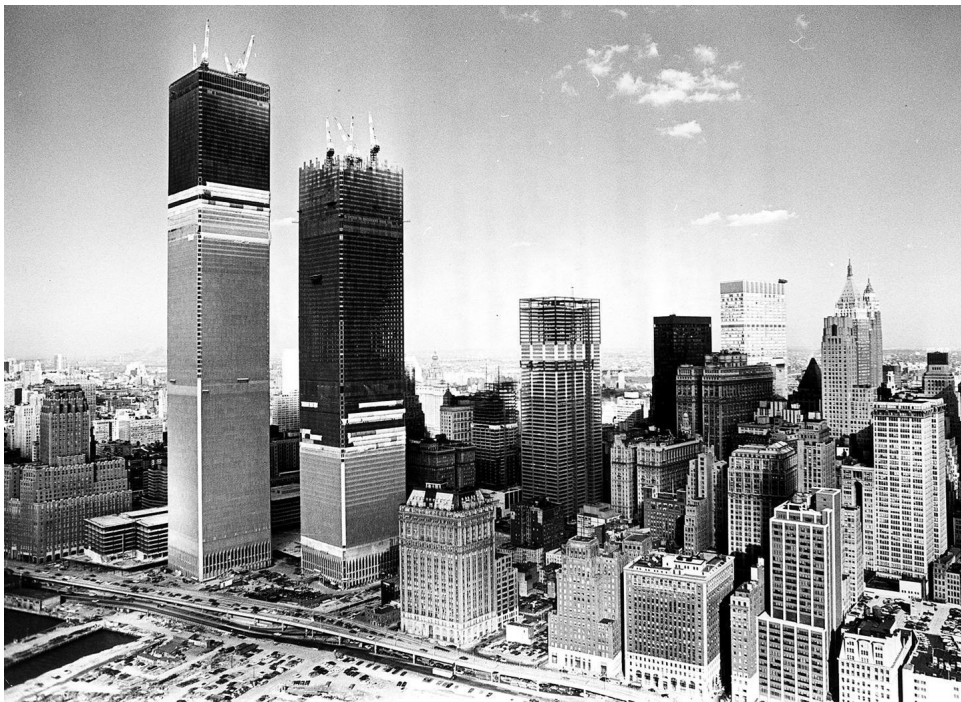
Fig. 1.4. Construction of the World Trade Center [14]
