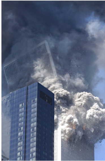
Fig. 1.5. Collapse of the North Tower [15]
