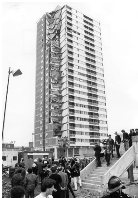
Fig. 1.1. Ronan Point collapse [4]
