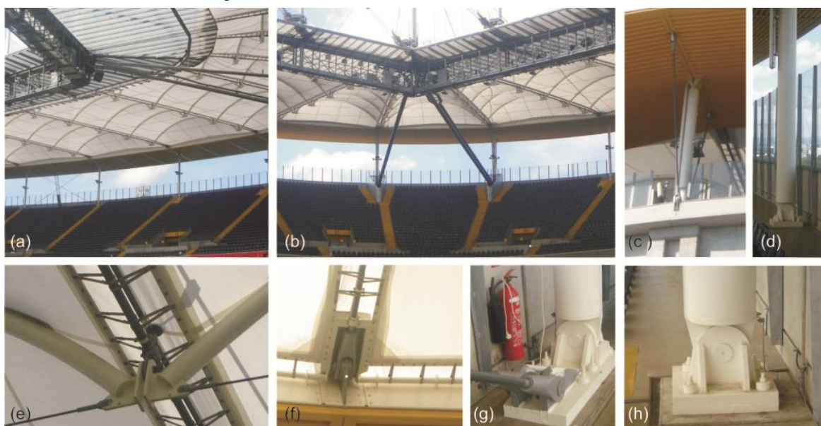
Figura 2.4-10 – New Waldstadion, Frankfurt/ Main
