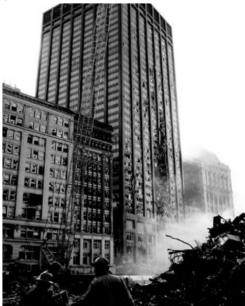
WTC debris, Bankers Trust Building, 2001
