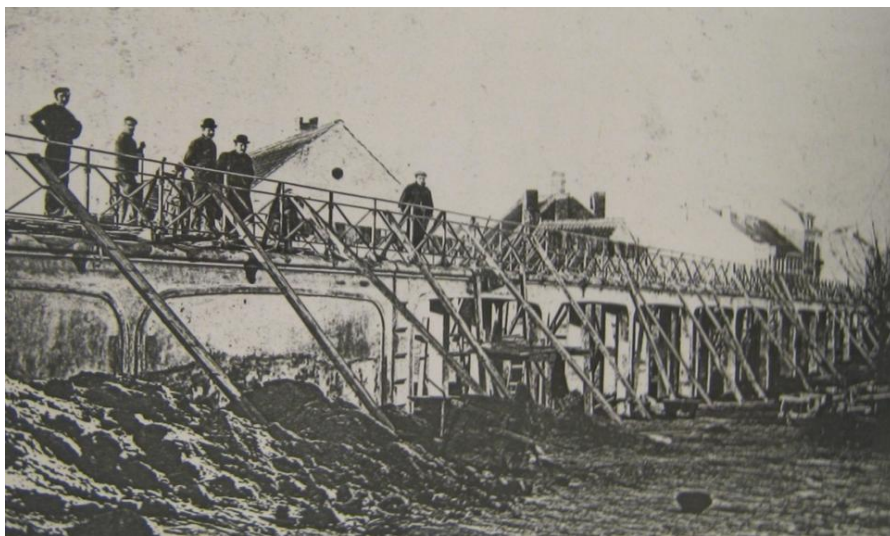
Testing to failure of an early reinforced concrete beam (1904) - span 6 m
