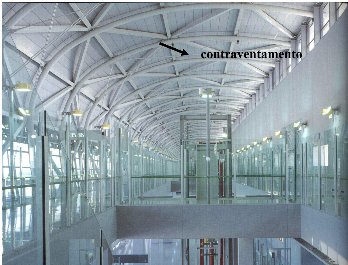
FIGURA 3.9 - Contraventamento horizontal FONTE – KANSAI INTERNATIONAL AIRPORT, 1994.
